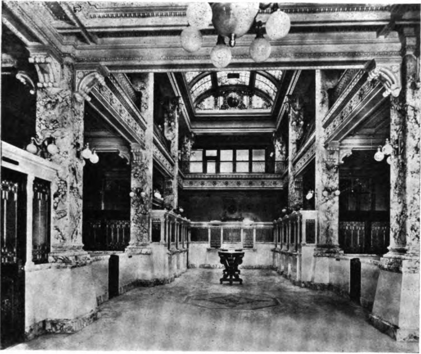
A View of the Main Lobby
